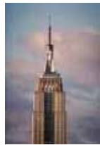
Empire State Building de Nova York
